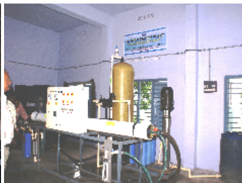
Inauguration (extreme left) of 2500 LPH plant was setup in partnership with DST and Rajasthan State Science and Technology, September, 2010, Theekariakalan village, Nagaur-Dist., Rajasthan. Feed :10,000 ppm; Product water :300 ppm (Left) and Siripuram village, Nalgonda district, AP (August 2009) 4000 LPH plant set up with DST and AP State Council support for removal of brackishness and fluoride (Right)
